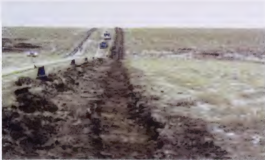
Photo 32 Partial sod salvage in shallow topsoils
